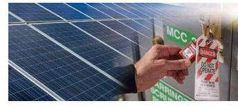
4. Once you have verified there is no voltage in each component, apply the lock and tag to each component with the worker's name, date, energy sources, isolating devices, magnitude of stored energy, and work being performed.
