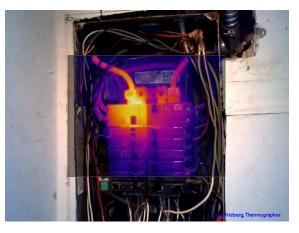
Heat can often be a sign of electrical problems such as loose, over-tightened, corroded connections, or other component failures. These areas can be seen easily with a thermal image, allowing qualified individuals to correct problems before significant damage or major failure occurs.
